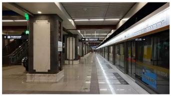
2. Avoid the passengers were sucked by strong negative pressure cause by the upper and lower high-speed passenger train passing and generated tragedies. Since the installation of platform screen doors there is no need to set the safe distance yellow lines, which can free up some space for the subway platform.
